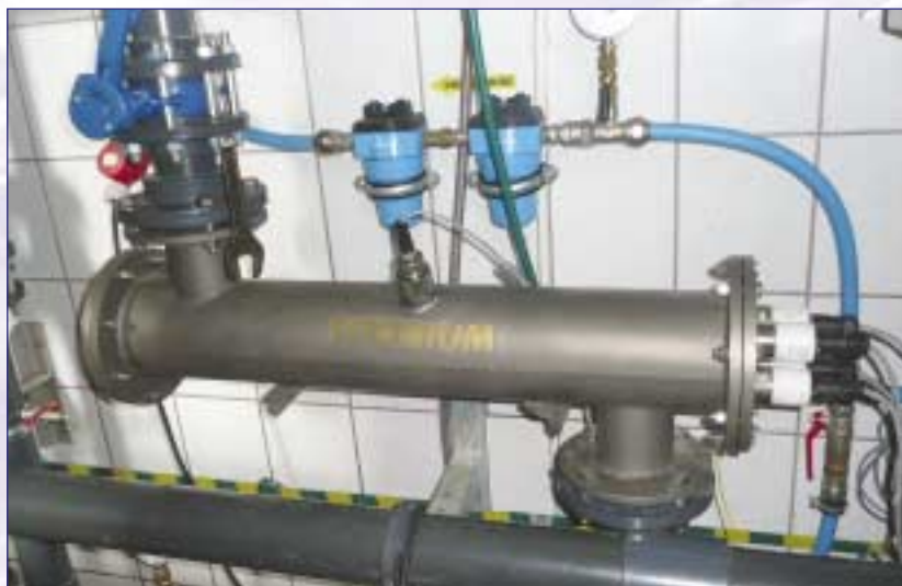
Typical Titanium AOP installations
